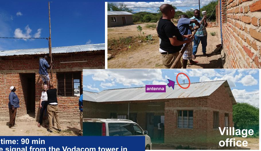
Installation time: 90 min catching the signal from the Vodacom tower in Migoli (~10km away)
